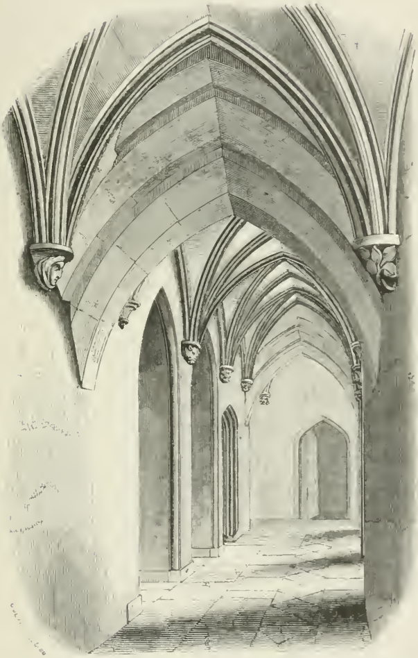
RUINED PASSAGE LEADING FROM THE HALL TO THE CHAPEL BROUGHTON CASTLE OXFORDSHIRE
